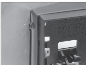
Insert the Angle Adapter into the hole and align the screw holes with the holes in the Angle Adapter. It may be necessary to relieve the panel to provide space around the screw heads on the left side of the Angle Adapter.
