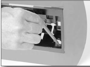
Remove one edge clamp at a time and mark the position of each hole with a pen. Use a circular motion to mark the outer edges of the hole. This will make it easier to determine the exact center. Do this for all four holes, replacing the edge clamps as you go.
